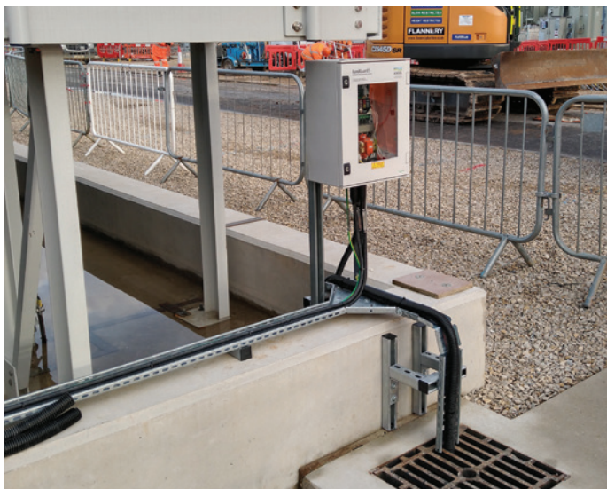
Bespoke special-build installation using National Grid specification enclosures, designed to incorporate a glycol loss detection system
